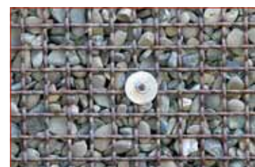
Joe Bellomo's street-front fence is made of gravel dropped between layers of steel mesh.
